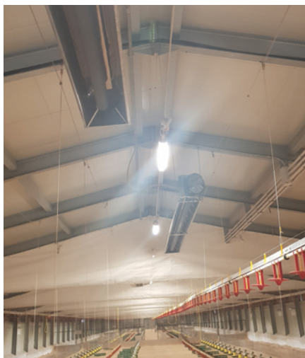
Fig. 9. Use of large infrared brooders.
