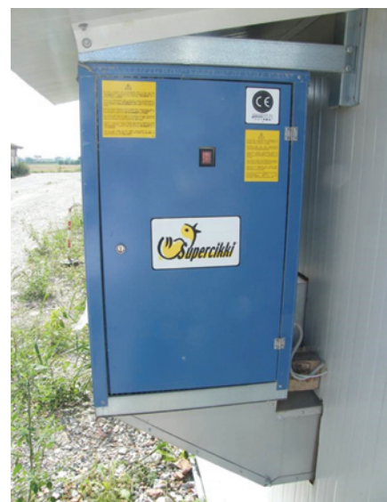
Fig. 6. Exterior hot air blower.
