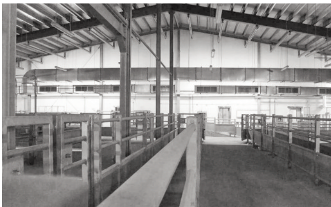
Waiting area with air-conditioning for livestock.
