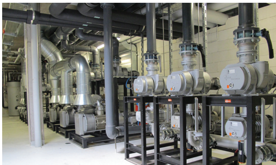
Central vacuum unit for the supply of vacuum to 10 packaging lines at Schwarzwaldhof. 'Pfefferbeisser' is one of Schwarzwaldhof's sausages speciality.
