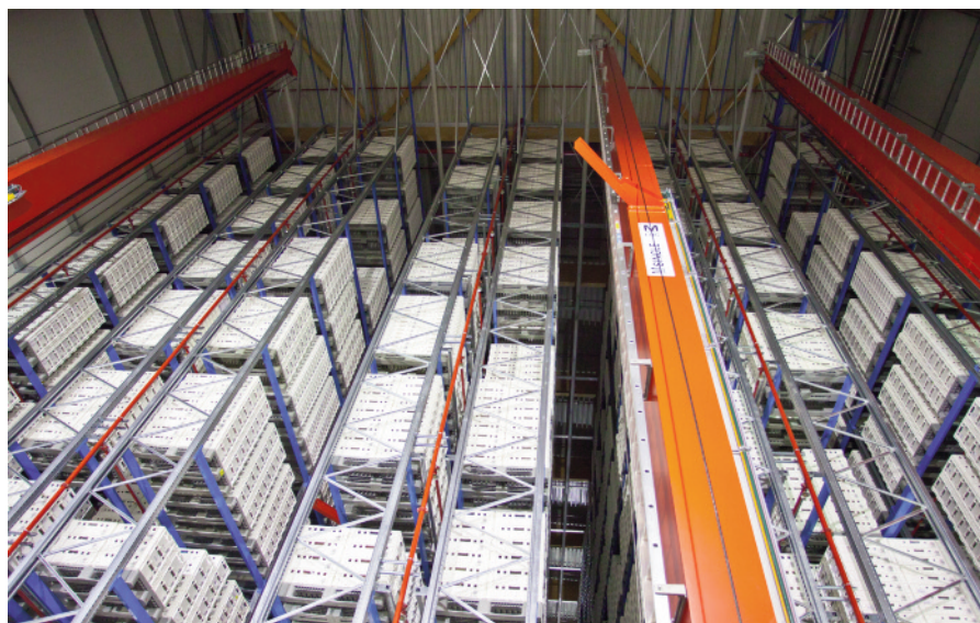
The IT system controls all stock entry, removal, and transfer processes of the high bay shelf storage with its 3,500 pallets.
