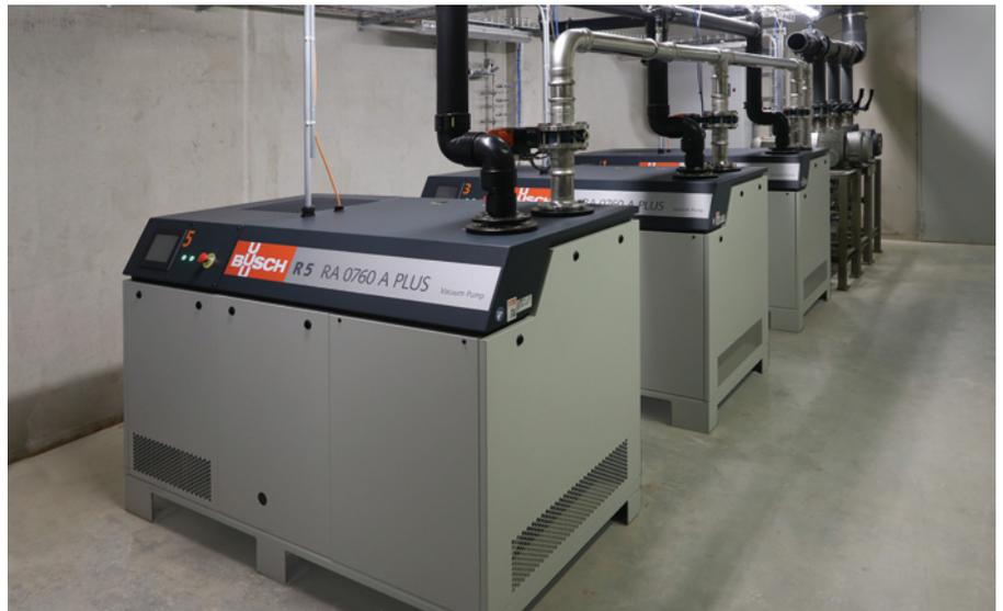
**Modern vacuum technology with the latest PLUS Master Control unit from Busch Vacuum Solutions offers efficient central vacuum supply according to actual demand.**
