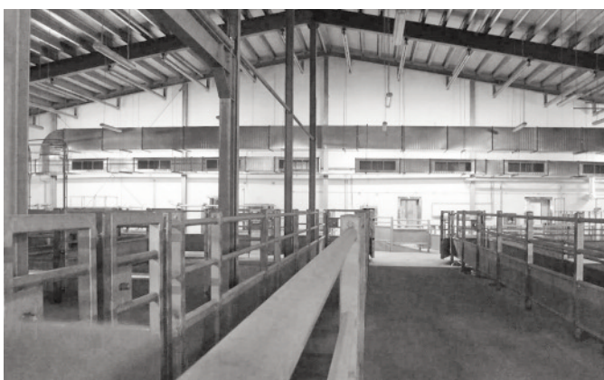
Waiting area with air-conditioning for livestock.
