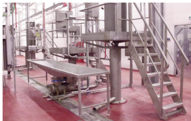
Trim platforms with pneumatic gun station for fat trims to fat line.
